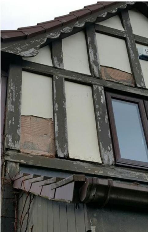
This image to the left demonstrates what can go wrong, in this instance the timber has been planted onto the external masonry cavity wall and the panels rendered in between. Movement in the timber then leads to water ingress behind the render and premature failure of the render system.
